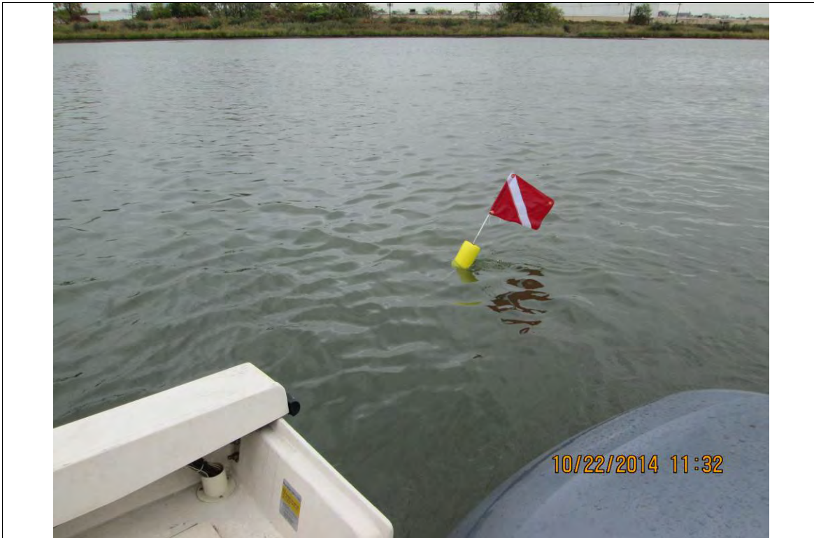
Photo 5: Buoy-marked plate location for cap thickness verification in subtidal area
